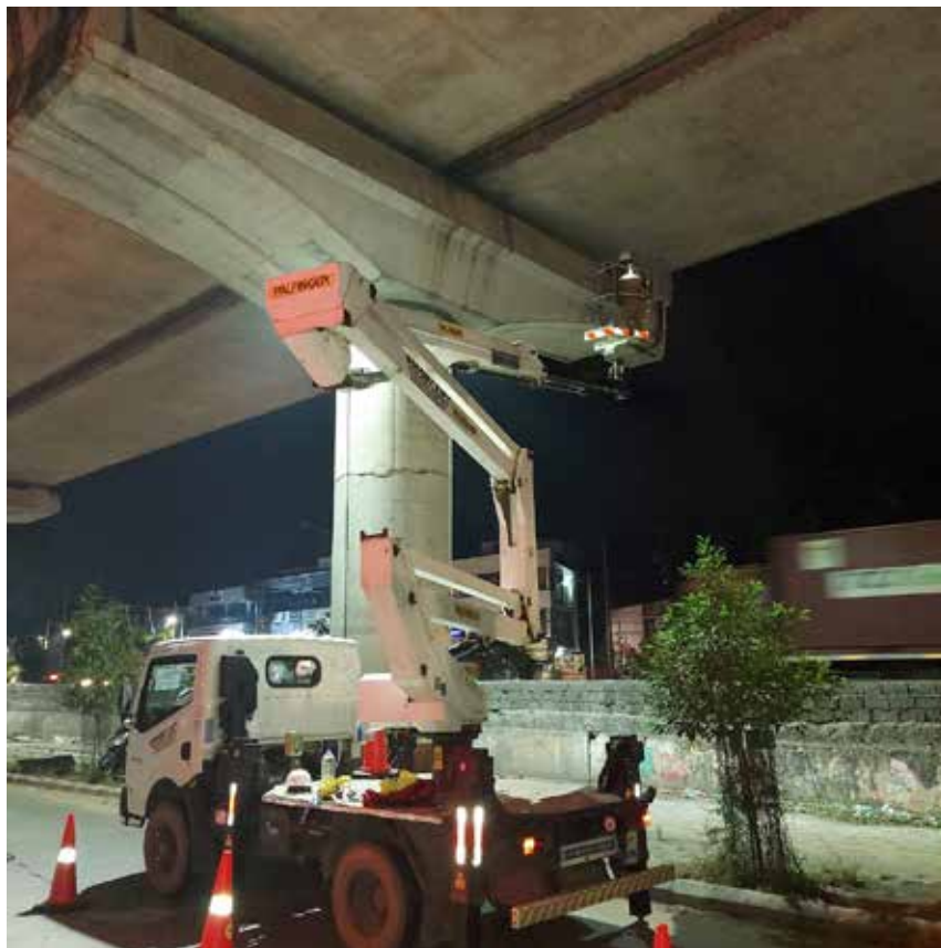
Conducting Study on Operation & Maintenance Processes of Kochi Metro Rail Limited – Field Study Inspection of Duct
