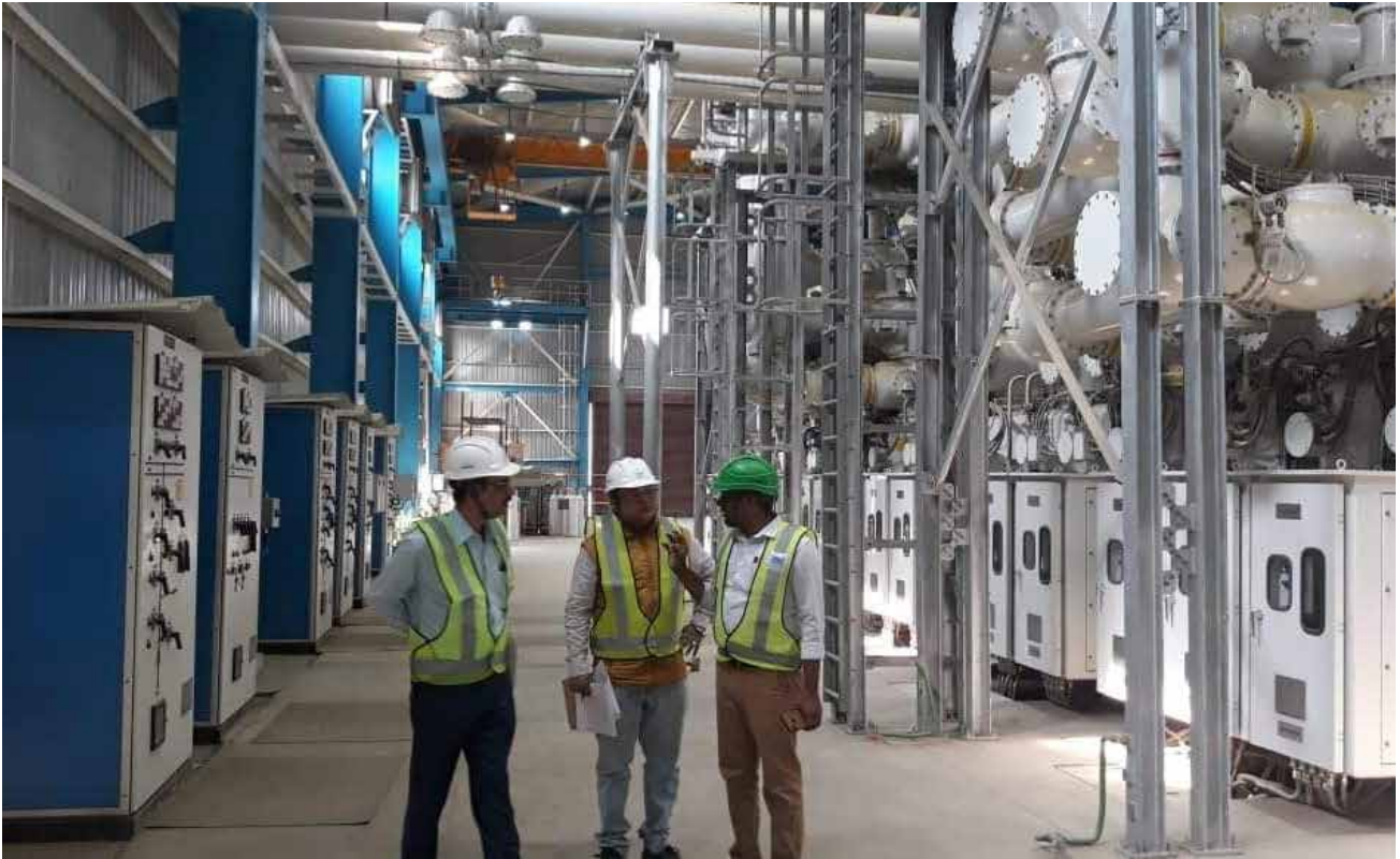
External Safety Audit at NTPC-Khargone
